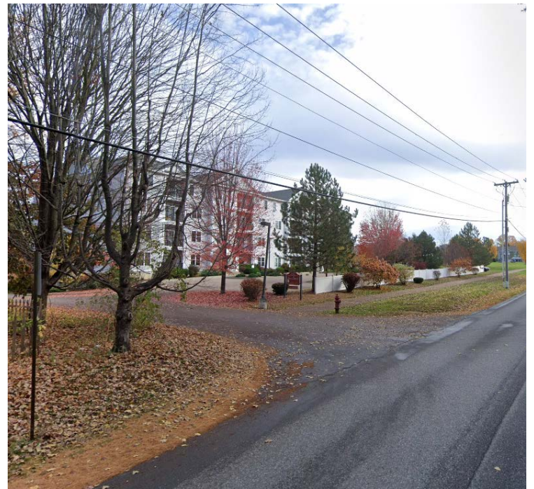
Start of Existing Shared Use Path at Farm Stand Apartments
